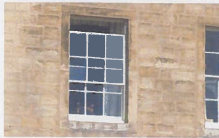
Vertical sliding sashes
