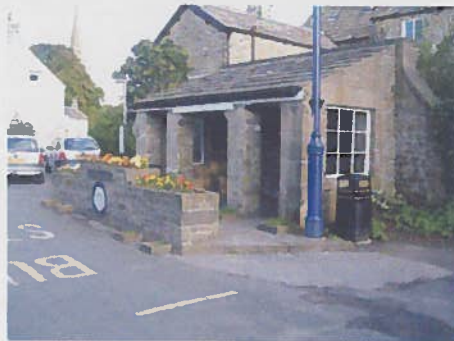
The southern side of Little Market Place is an untidy mix of the rears of properties, street furniture, shelters and hard landscaping.
