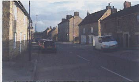
Properties 14-18 Park Street in the right hand foreground display a shallower pitch from the late-eighteenth century, while following building (No 24) clearly dates from the seventeenth century, both are of local stone with ashlar dressings and graduated stone slate roofs.
