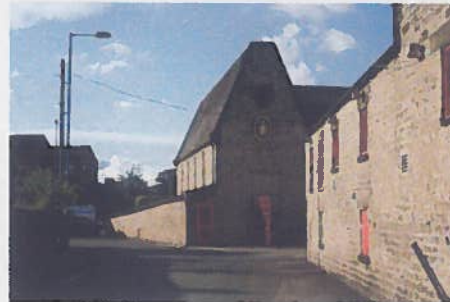
Theakston's complex of buildings was purpose-built as a brewery and maltings and the unusual roof forms reflect functional uses within the buildings
