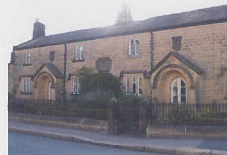
2-8 Swinton Terrace, the almshouses, although presently unlisted are without doubt 'landmark' buildings within Masham. Formalised front gardens and decorative railings demarking the boundaries are not common features in Masham.
