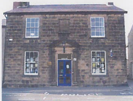
The Community Office, Little Market Place: a late eighteenth century building of coursed, dressed stone with a Welsh slate roof. (Grade II listed)
