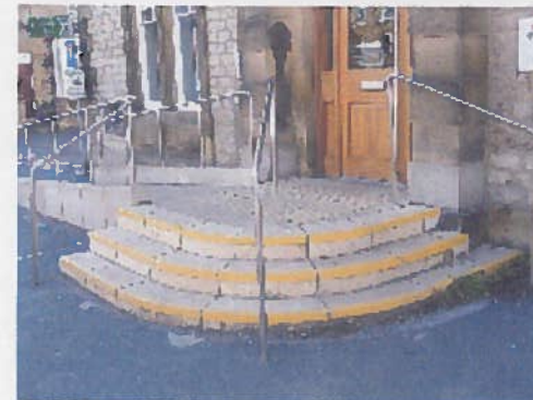
Inappropriate detailing and materials can have a significant effect on the special character of a place.
